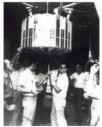
**Figure 4.** Paul J. Dick preparing to install the SNAP-3B7 RTG on the Transit 4A satellite, June 1961.
