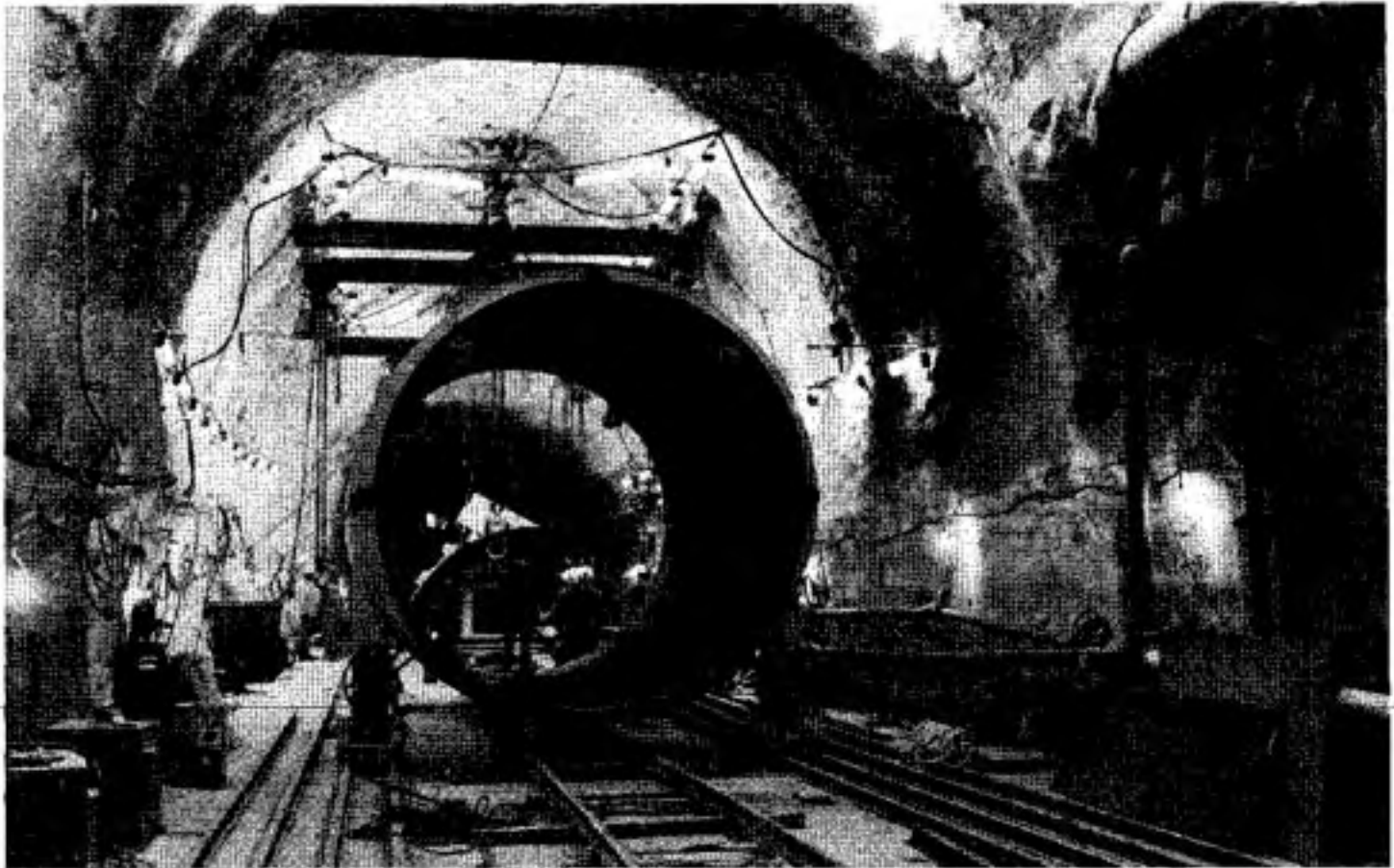
Figure 2 23 Tunnel for weapons effects test. Huge tunnels are drilled into Rainier Mesa at the Nevada Test Site, the primary area for weapons effects tests. Sections of pipe are joined together to encase test chambers, materials, and components. The biggest pipes used to
