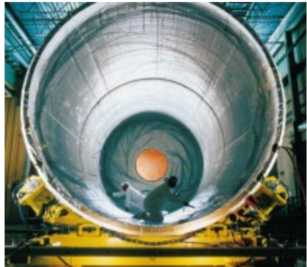
Figure 3-18: Installation of lining inside a motor case.
