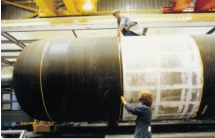
Figure 3-20: Installation of internal insulator prior to motor case filament winding operation.
