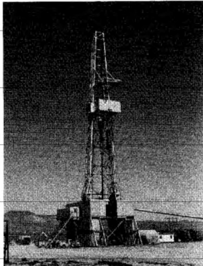
Figure 2 15 The IDECO 2500 Drill Rig. This 2,000 horsepower diesel electric rig is capable of drilling holes 72 to 140 inches in diameter to depths of 4,000 feet. The rated capacity of its 158 foot Pyramid Mast is 1,400,000 pounds.
