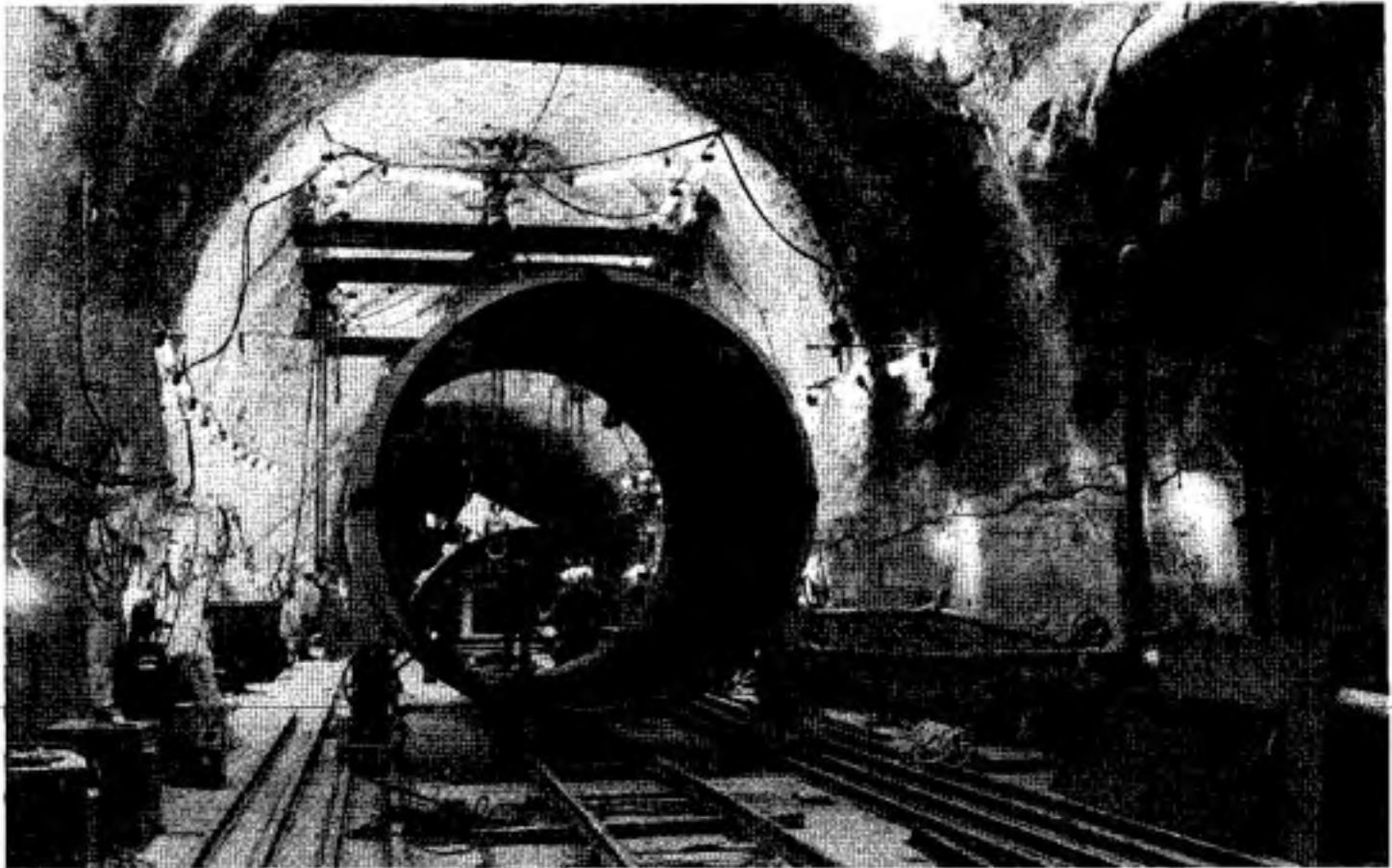
Figure 2 23 Tunnel for weapons effects test. Huge tunnels are drilled into Rainier Mesa at the Nevada Test Site, the primary area for weapons effects tests. Sections of pipe are joined together to encase test chambers, materials, and components. The biggest pipes used to
