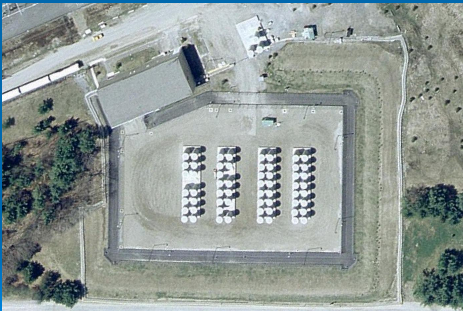
Maine Yankee Dry Cask Storage Installation
