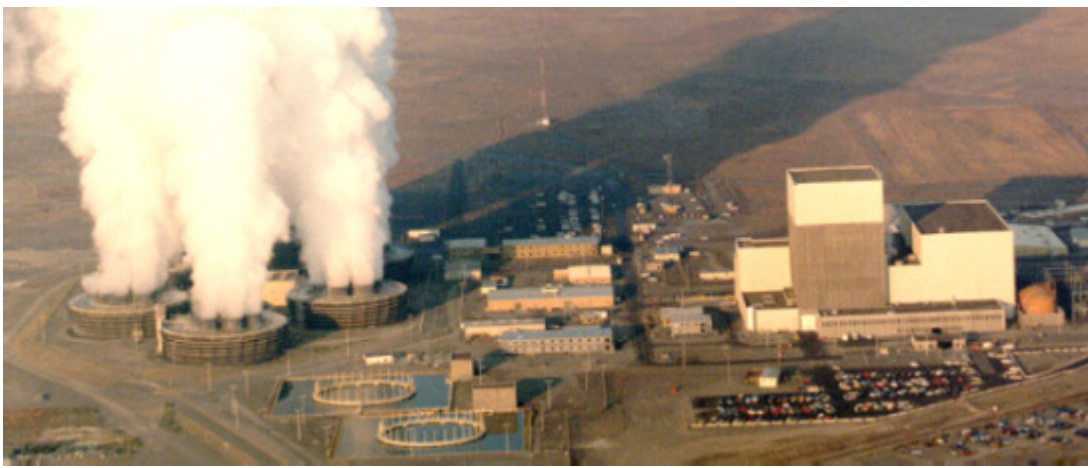
Six large cooling towers serving Washington Public Power Station's Unit -2 (3323 MWt) at Hanford Reservation, Washington [46 28 17N; 119 19 59E].
