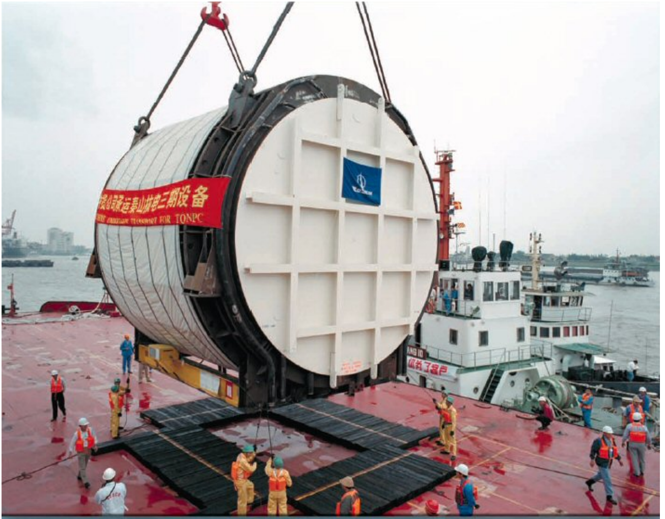
CANDU-6 reactor vessel in transit.
